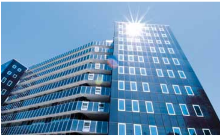
Enzian Tower - PV Fassade, Bozen
